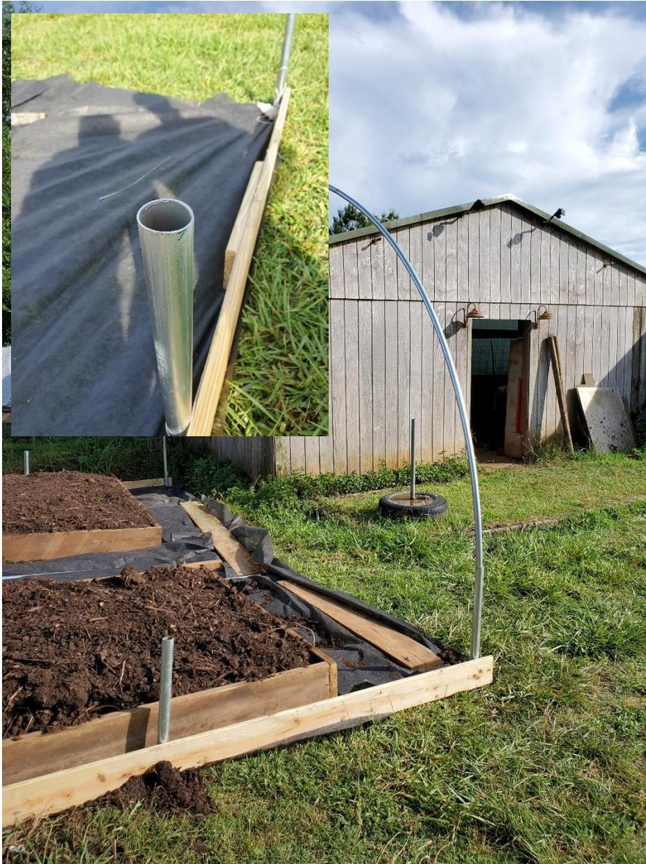
Once the corners and side posts are in the ground, trim all mushrooming off with a hacksaw or an angle grinder with a cut off wheel (*much* faster, but wear eye protection...). Then, locally source some 5/4 decking and use 2" pipe straps to attach it on the *outside* of your posts at the ground level. This will provide a surface you can attach plastic to later on.
