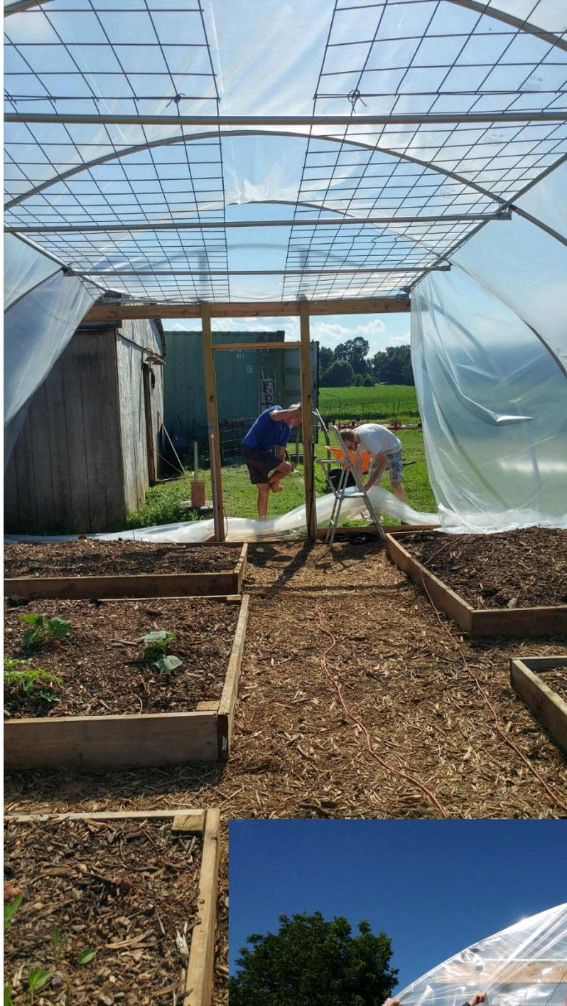
We laid the end sections along each end and pulled the center (top) section down one side. We began by attaching the one side, then pulling the plastic over the top and simply weighting it on the opposite side.
