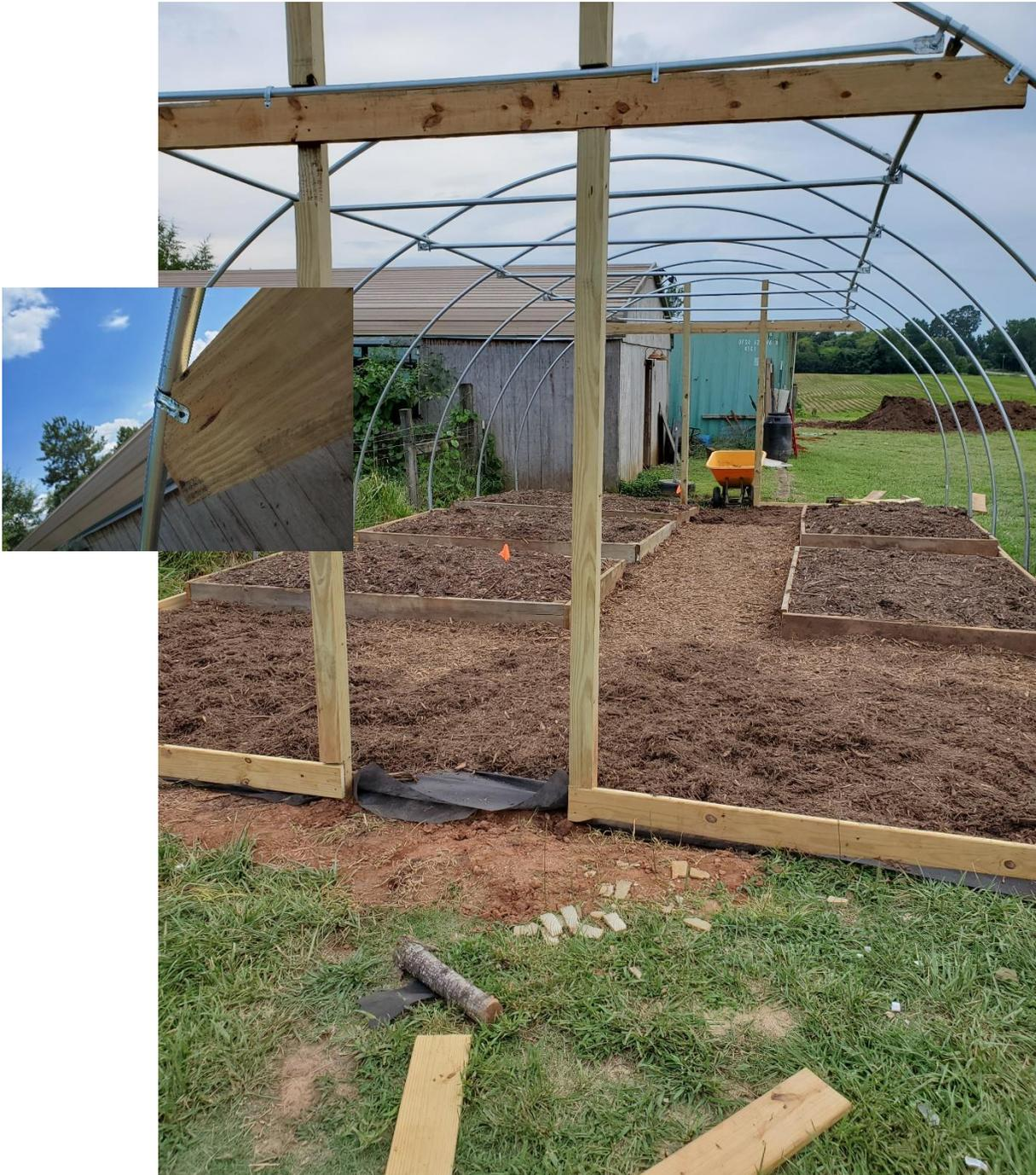
We used 4" x 4" x 12' treated posts to frame our doorway with a top rail that is a 2" x 6" x 12' brace. We notched the posts, see pic below, for the brace. Later, we will put an upper brace where the top of the door will be. Bent and drilled pipe straps, as in the pics above, were used in four places to secure the cross brace on the hoop to the 2 x 6. These pics were taken after the purlins were installed
