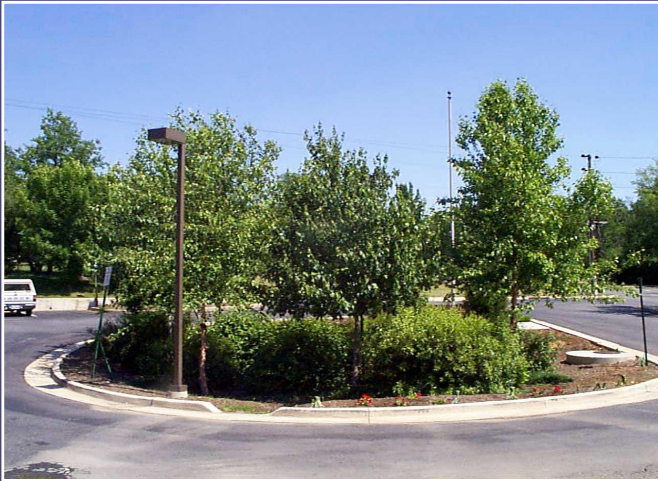
Parking lot planter islands (bioretention)
