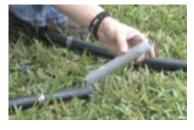
1. Attach all of the poly hose together by inserting a 8" long piece of 1/4" CPVC into the open end. It should be very tight and hard to insert.
