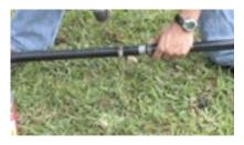
5. Tighten with hose clamps and repeat as necessary so you have a long 500" length.
