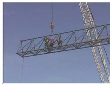
To rise to its maximum height, the crane *grows* itself one mast section at a time! The crew uses a **top climber** or **climbing frame** that fits between the slewing unit and the top of the mast. Here s the process:
