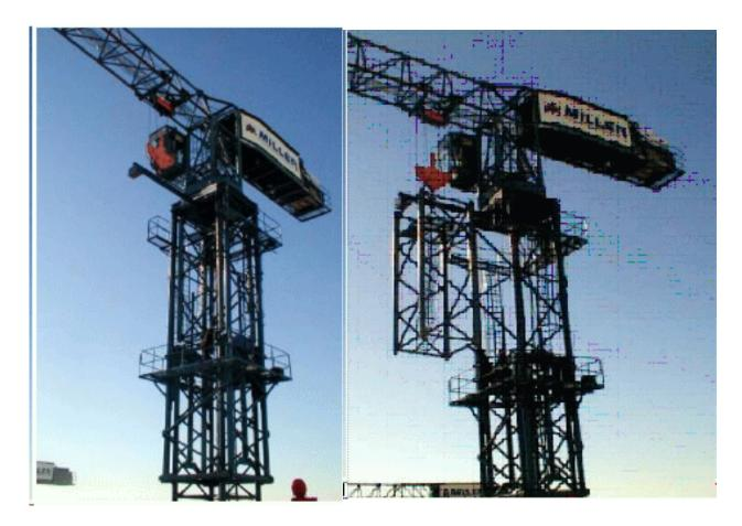
Once the building is finished and it is time for the crane to come down, the process is reversed -- the crane disassembles its own mast and then mobile cranes disassemble the rest.
