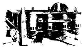
The power poant the Wright brothers developed for their 1903 Flyer. It was a four-cylinder piston engine weighing 179 pounds, producing 12 horsepower at 1,090 revolutions per minute. The engine drove 2 propellers.
