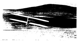
Wilbur Wright in same glider making a right turn. This glider is the first winged vehicle capable of full control in roll, pitch, and yaw axis.
