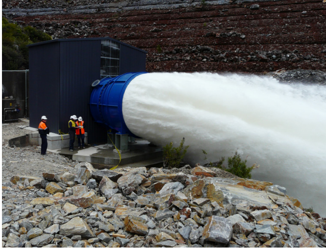
Rowallan Dam/Hydro, Tasmania, Australia—One Howell-Bunger® Valve (72") with stationary hood and venting
