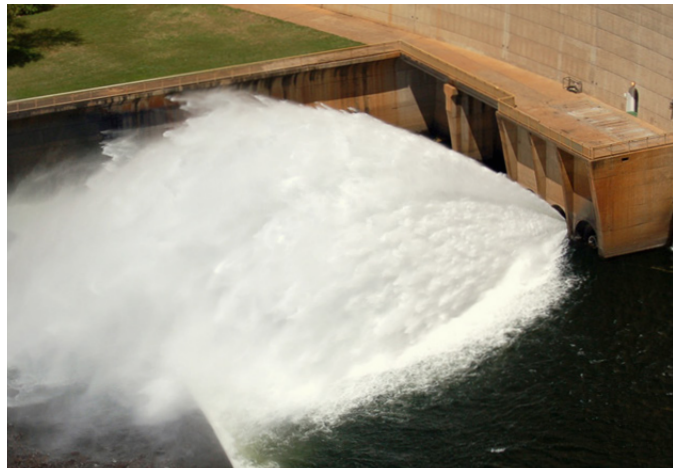
Jozini Dam, South Africa - Three Howell-Bunger® Valves (72"), half-submerged discharge with head of 262'
