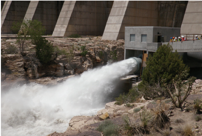
Pueblo Dam, Colorado, USA—One Howell-Bunger® Valve (60") with stationary hood and One Rotovalve® Cone Valve (60")
