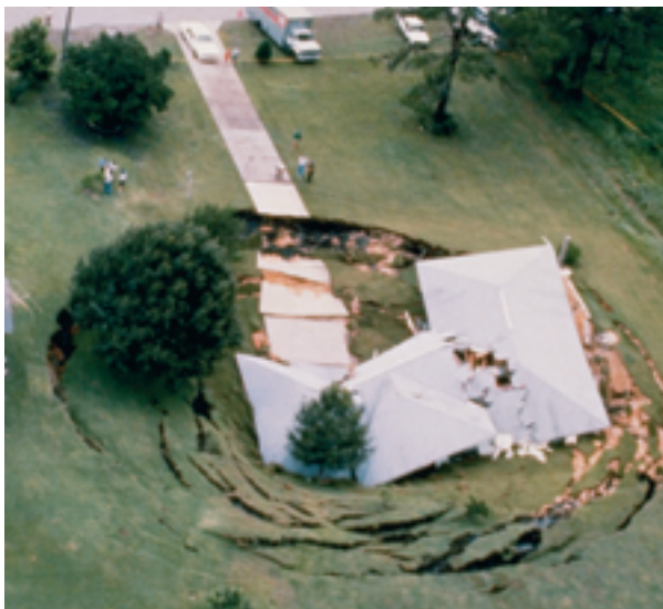
Figure 24 This small sinkhole formed suddenly in 1991 when the roof of a cavern collapsed. It destroyed this home in Frostproof, Florida.
