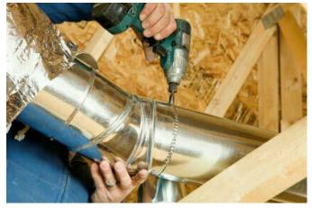
All new duct work with connections are sealed and tested. All ducts running outside of building will be insulated.
