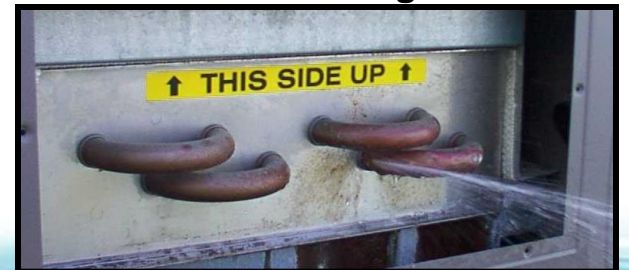
Freeze Damage
