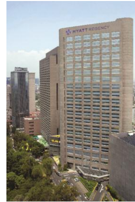
Hyatt Regency Mexico City 755 Rooms
