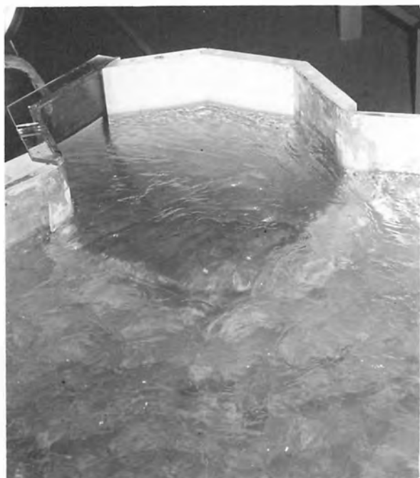
C. Gate 75% Open. Q = 300 cfs. Head at gate = 51.0 feet
