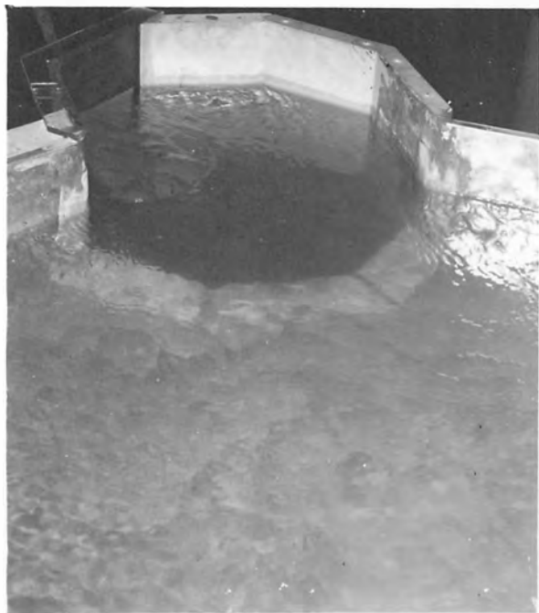
D. Gate 100% Open. Q = 300 cfs. Head at gate = 39.6 feet.
