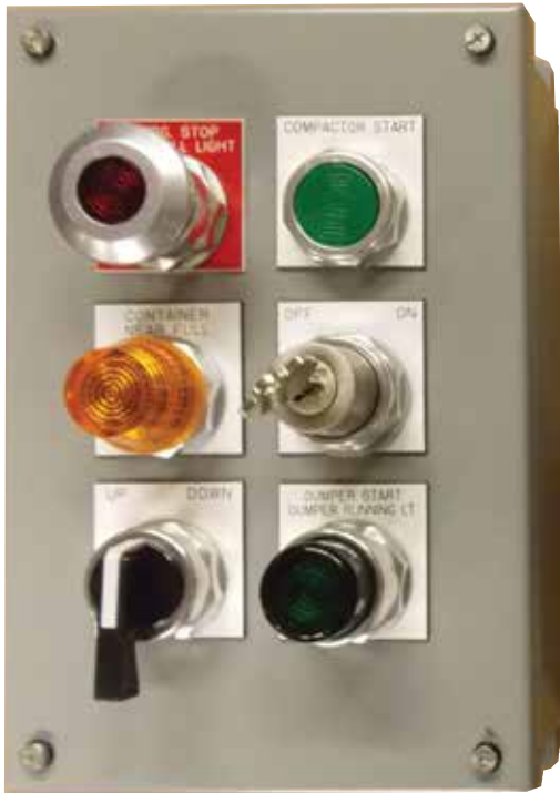
Automatic Cycle with Advance Warning Light and Dumper Remote Control Station
