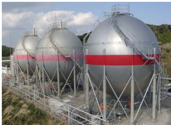
H-II rocket fuel hydrogen storage tank
