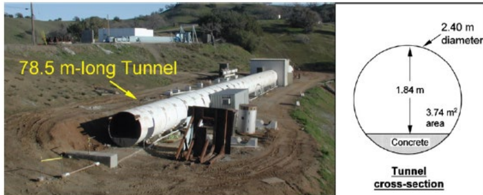
Figure 4: SRI Corral Hollow Experiment Site Tunnel Facility (from [40])
