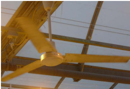
Figure 14. Paddle fan to increase vertical air movement and therefore evapotranspiration. This is important for the prevention of tipburn. A 17 mol/m 2 /d DLI target has to be matched with sufficient downward air flow to prevent tip burn. Without the air flow, we were not able to go over 12 mol/m 2 /d.
