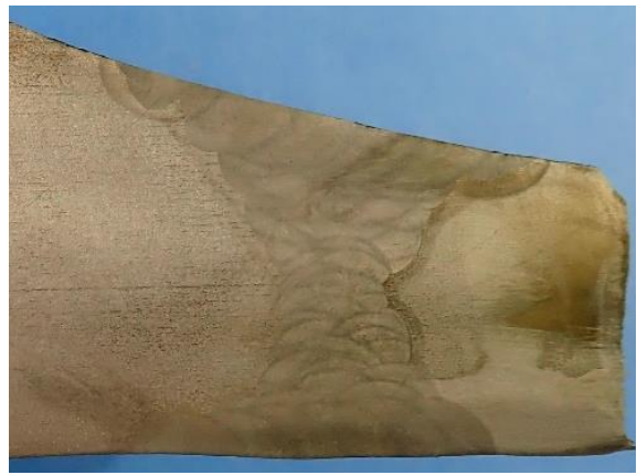
b. Weld profile near top of fractured side plate.
