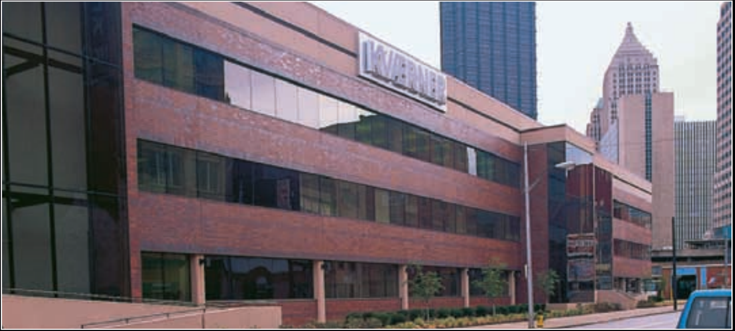
Liberty Plaza – Pittsburgh, Pennsylvania Medium Ironspot #46 – 1/2" x 3 5/8" x 11 5/8" and Dark Ironspot – 1/2" x 3 5/8" x 11 5/8" accent
