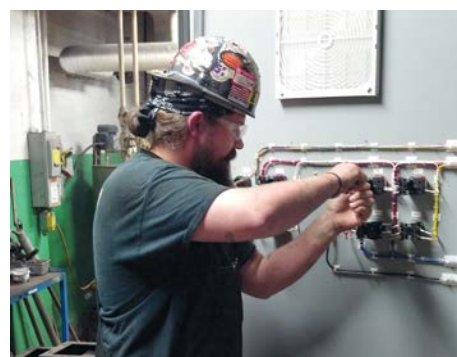
Local 557 member Ben Small, working for Nelson Electric, terminates a push button for a variable-frequency drive at Nexteer Automotive in Saginaw, MI.
