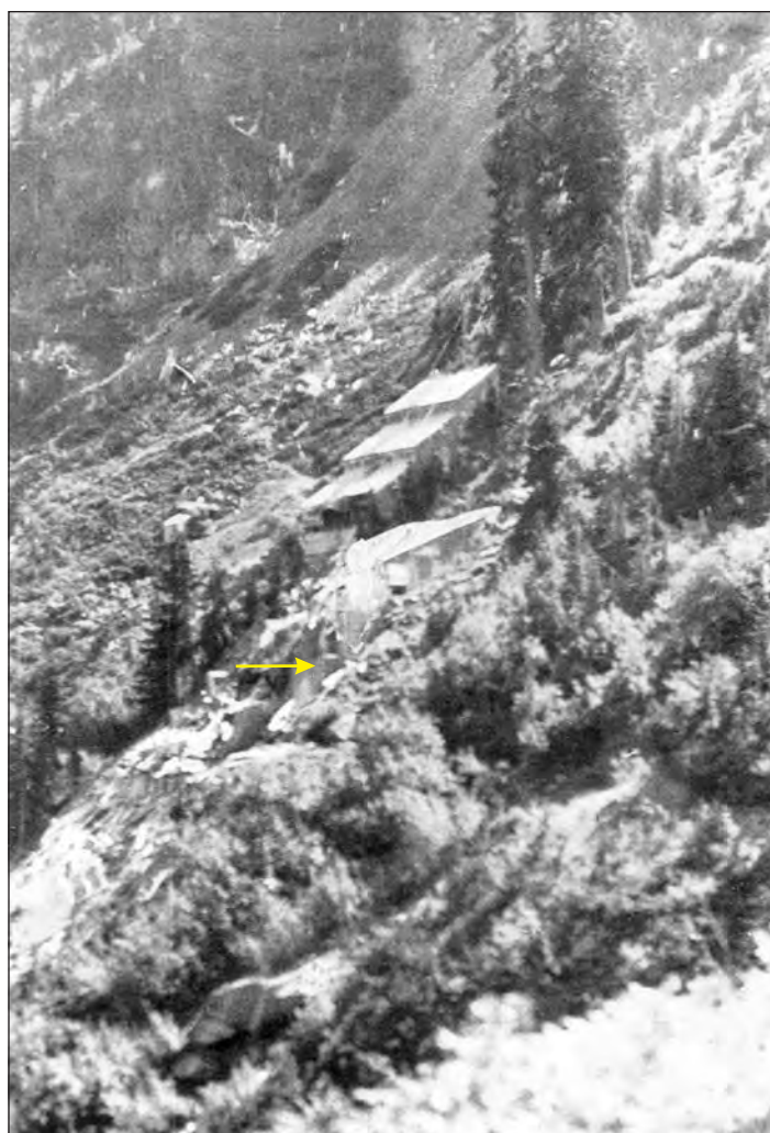
Figure 12. Flotation mill (arrow) destroyed by avalanche in foreground, relocated bunkhouse in background. Approximate date post-1924. Note trace of tramway cables in center. Photo courtesy of P. Jeffcott Collection.
