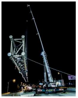
Thackray Crane Rental was called to help install a new highway signage truss over Interstate 95 in Philadelphia, USA. The lift required a 400 tonne capacity Liebherr LTM 1400.7.1
