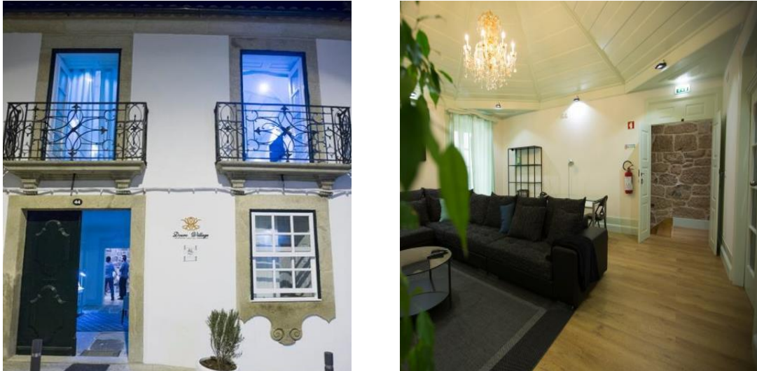
Figure 15 - Rehabilitated building - facade and interior
