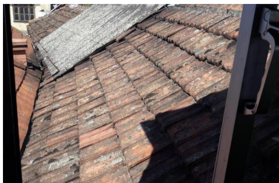
Figure 7 - Parasitic vegetation in Marseille tiles
