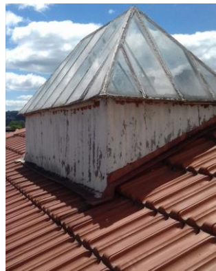
Figure 3 - Pitched roof with Marseille ceramic tiles and skylight
