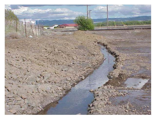
FIGURE 5-17. Seepage from Cut Bank
