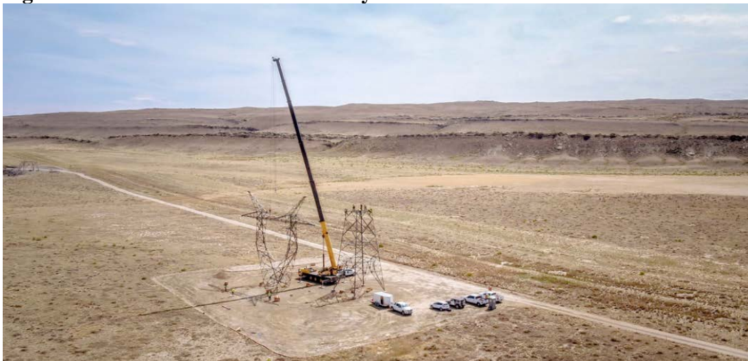
Figure 4.1 Construction of the Gateway West Transmission Line 187
