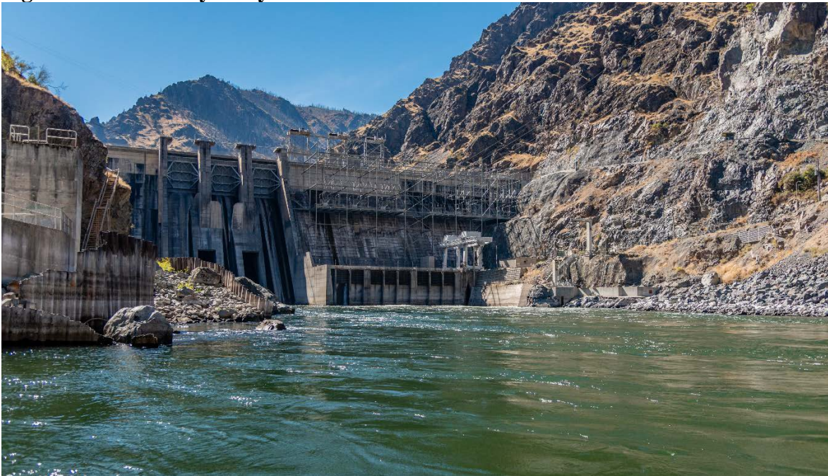
Figure 1.2 Hells Canyon Hydroelectric Dam 8
