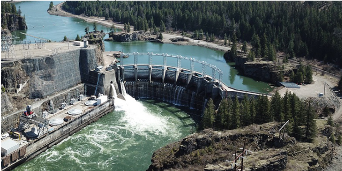
Figure 2.1 Cabinet Gorge Hydroelectric Dam on the Clark Fork River 117
