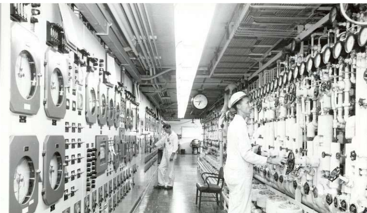
Figure 13. Main Processing Building, CPP-601, Operating Corridor. Source: INL Photo 55-1719.
