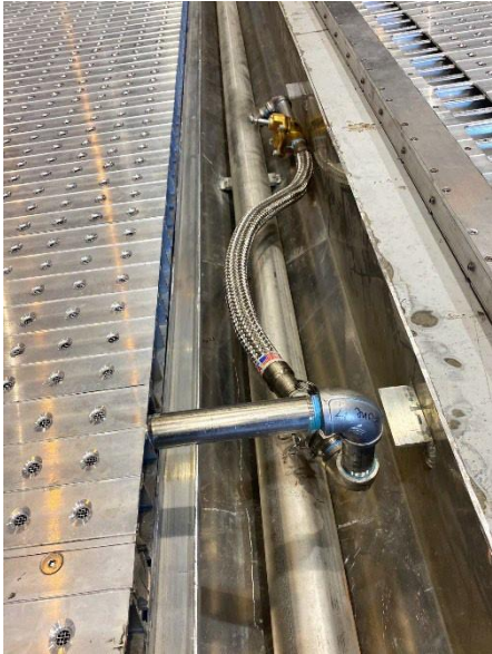
Water supply and discharge piping routed in prefabricated aluminum trenches
