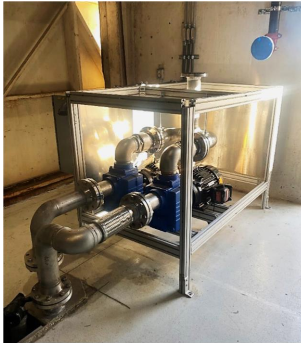
Figure 19: ILDFA pump skid installation during construction. External panels not shown.
