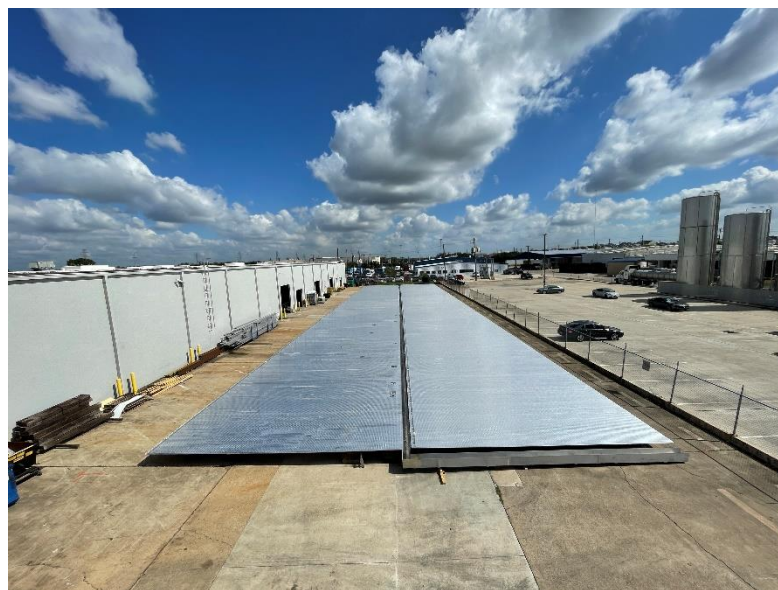
Figure 26: The flame detector testing was conducted on the ILDFA shown
