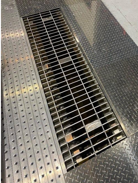
Trench covers with support frame and profile placement
