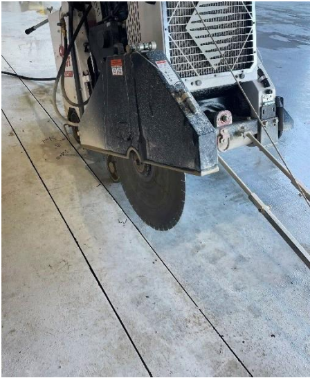
Cutting through existing concrete slab
