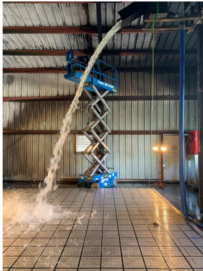
Figure 2-3: Spill device elevated to 15 feet using forklift for water testing. Flow rate shown is 400 gallons/minute.
