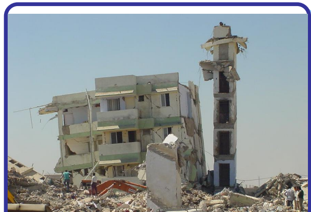
Figure 4: Deficient connection between slabs and vertical elements – collapse of an RC frame building during 2001 Bhuj (India) earthquake
