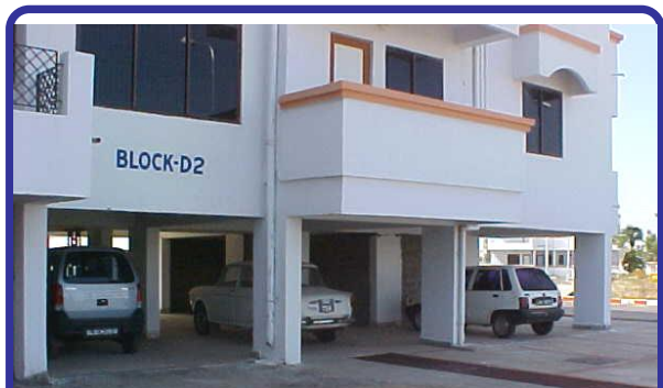
Figure 1: Ground storeys of reinforced concrete buildings are left open to facilitate parking – this is common in urban areas in India.
