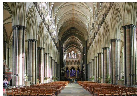
Figure 2: Rib Vaults and Pillars
