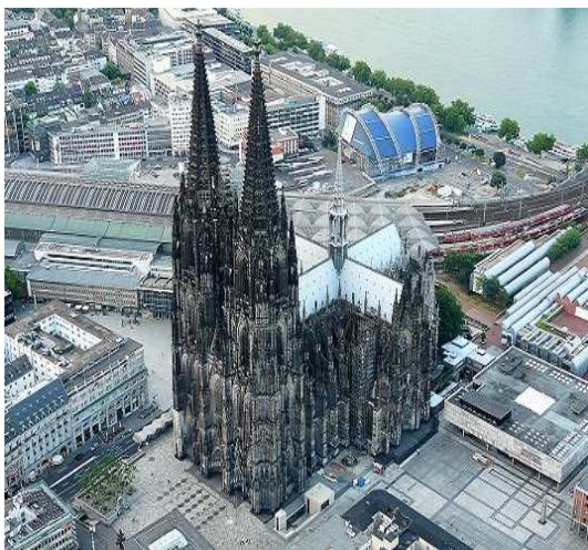
Figure 9: Spires, Several Supporting Structure around the Main Building
