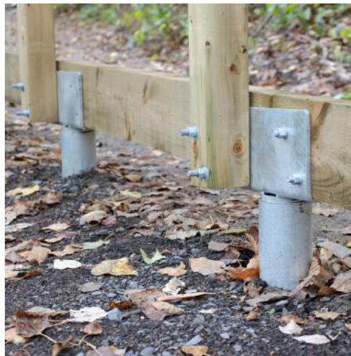
..... Left: Helical pile foundation .....
