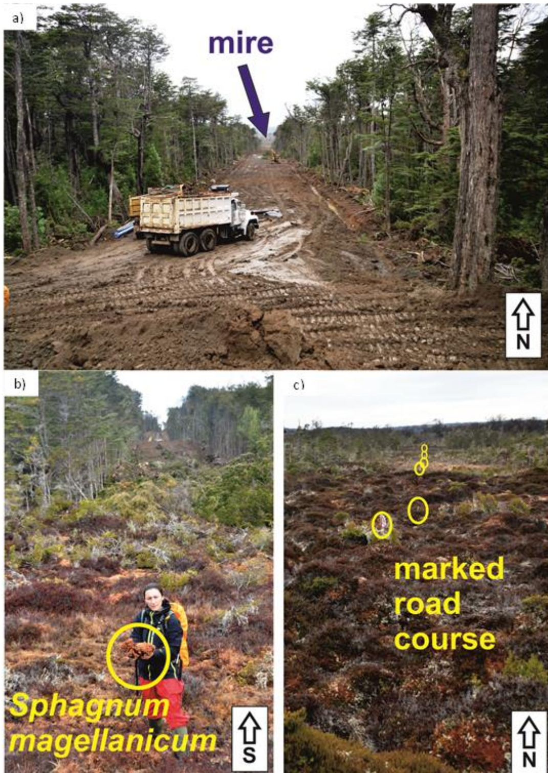
Fig. 2: a) Road currently constructed close to Seno Obstrucción with ca. 500 m through pristine forest until reaching a mire. b) Thick Sphagnum magellanicum cushions on the surface of the future road c) Currently not constructed but marked road course through a mire where peat thickness reaches >3 m.
