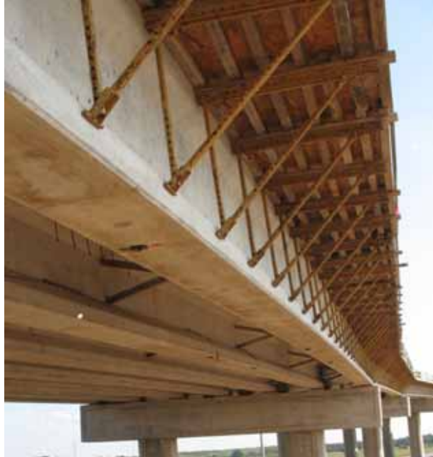
Figure 4.6: Overhang Brackets in Place
