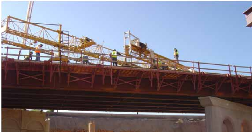
Figure 4.17: Lubbock Steel Plate Girder Bridge under Construction
