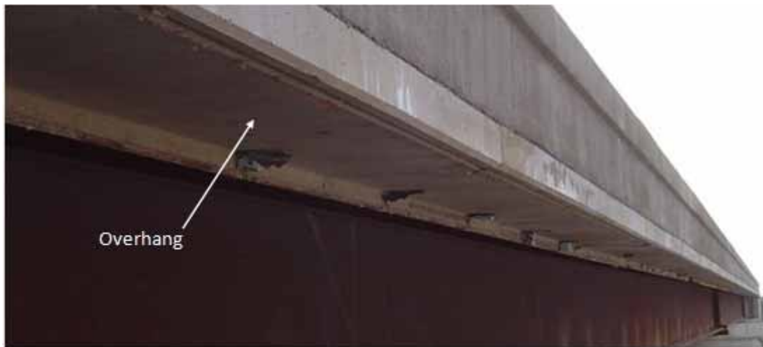
Figure 2.1: Bridge Deck Overhang
