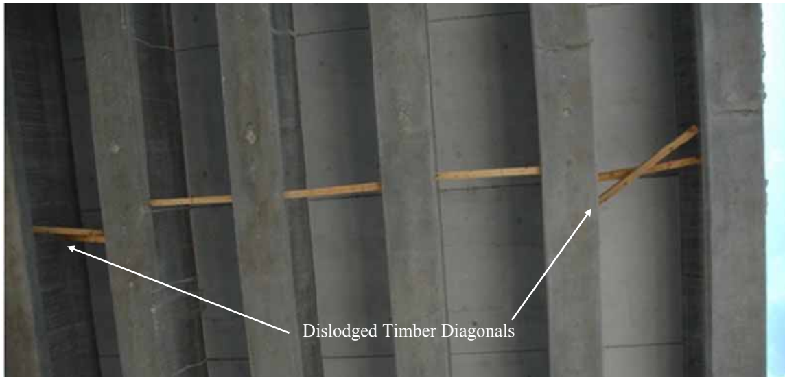
Figure 2.8: Effect of Twist on Timber Blocking
