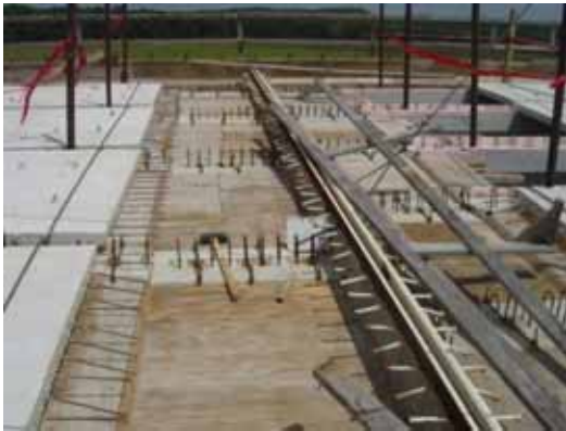
(a) Formwork for Thickened Ends
