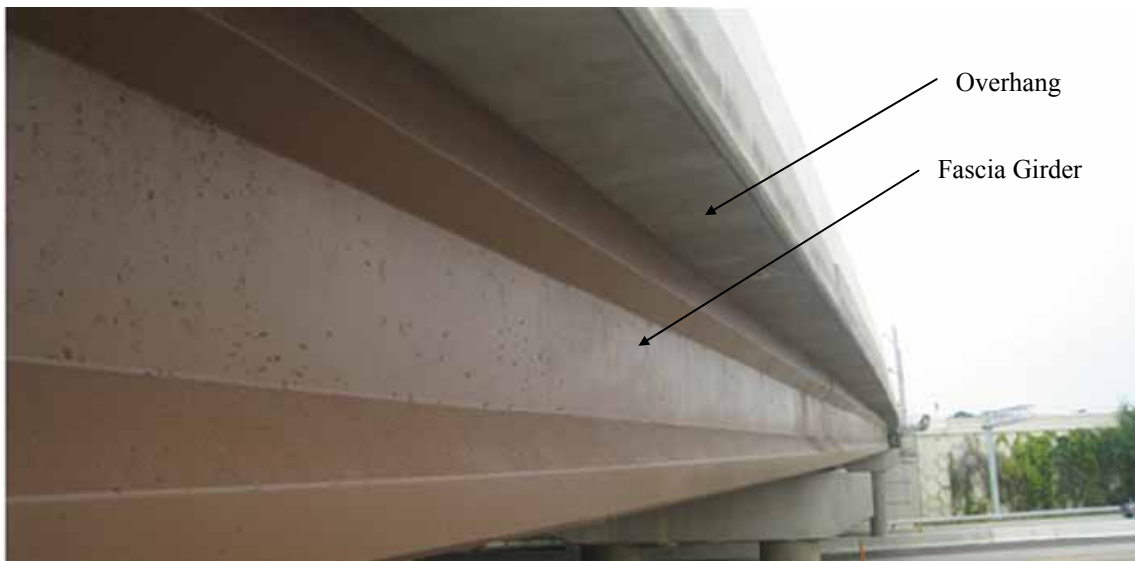
Figure 1.1: Overhang in Typical Concrete Girder Bridge
