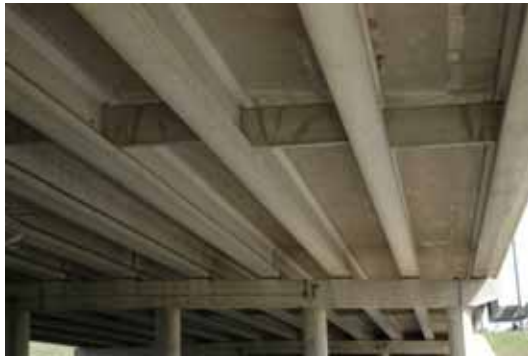
(a) Concrete Diaphragm
