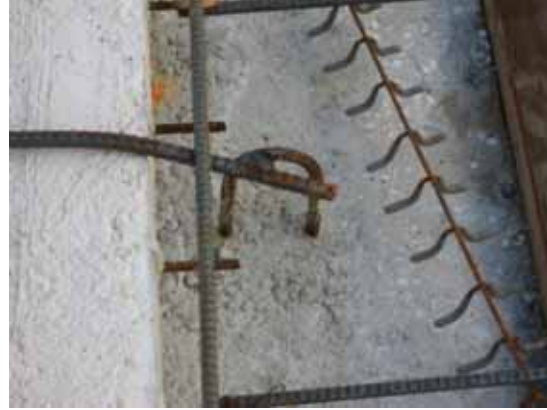
(b) Connection in Exterior Girder
