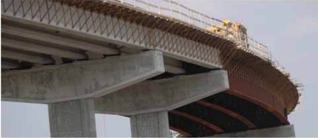
Figure 2.2: Overhang Brackets
