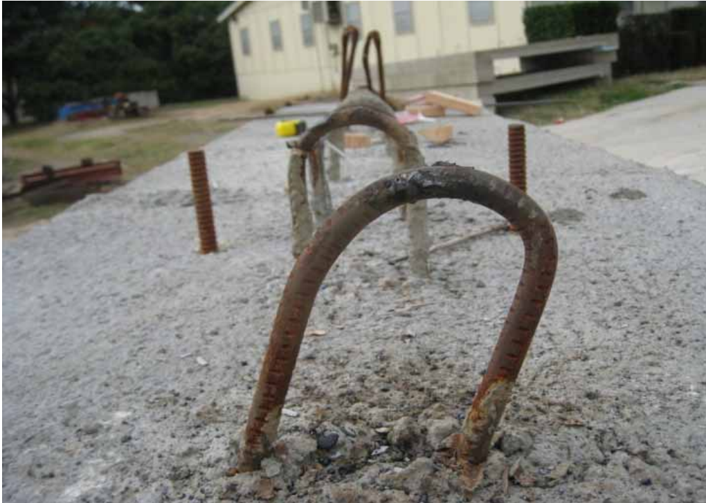
Figure 3.5: Permanent Deformation of R-bar after Removal of Load
