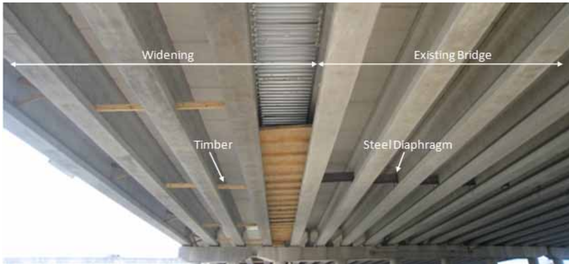
Figure 2.7: Advancement in Bracing for Concrete Girder System
