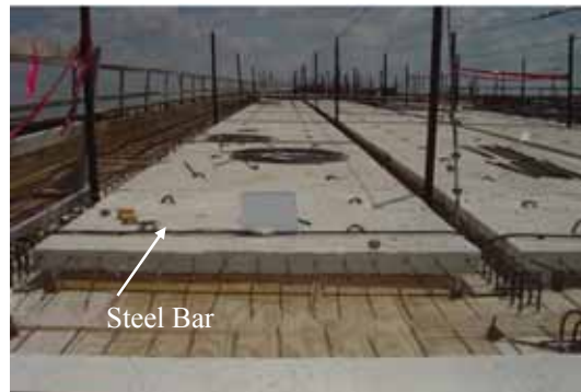
(c) Top Bracing Bar
