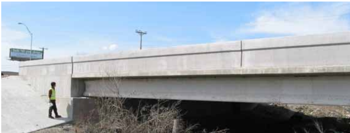
Figure 4.13: Hutto Concrete Bridge
