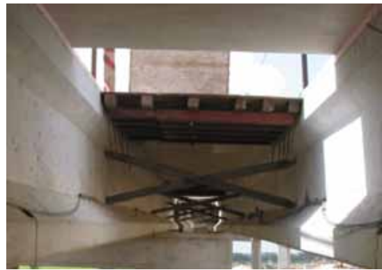
(b) Formwork for Drainage
