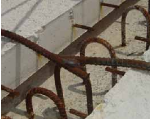
(a) Connection in Interior Girder
