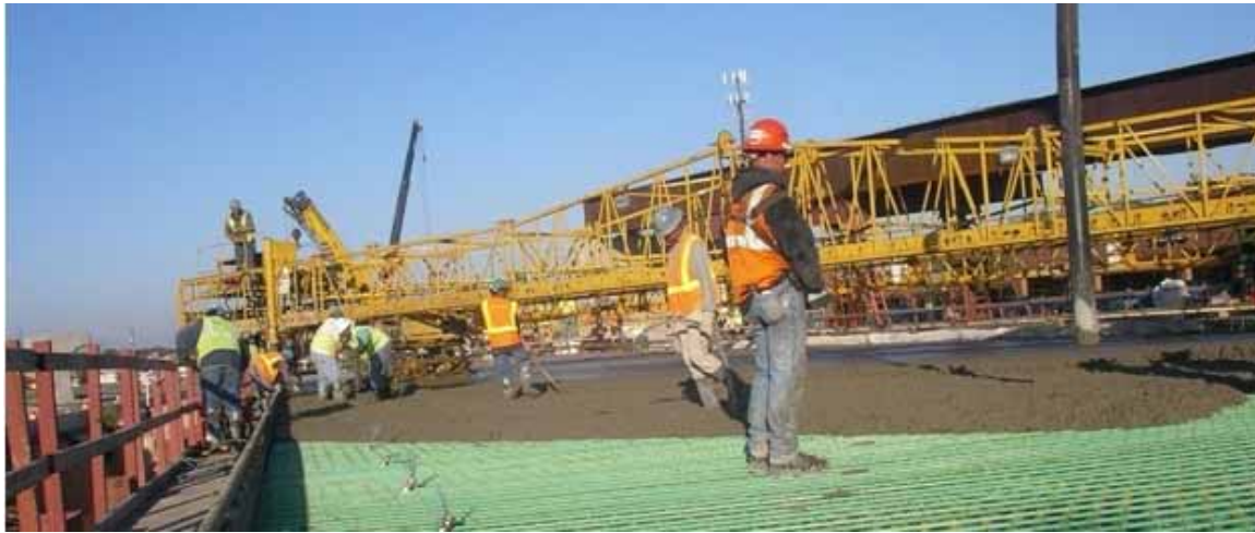
Figure 2.4: Bridge Deck Finishing Screed in Operation
