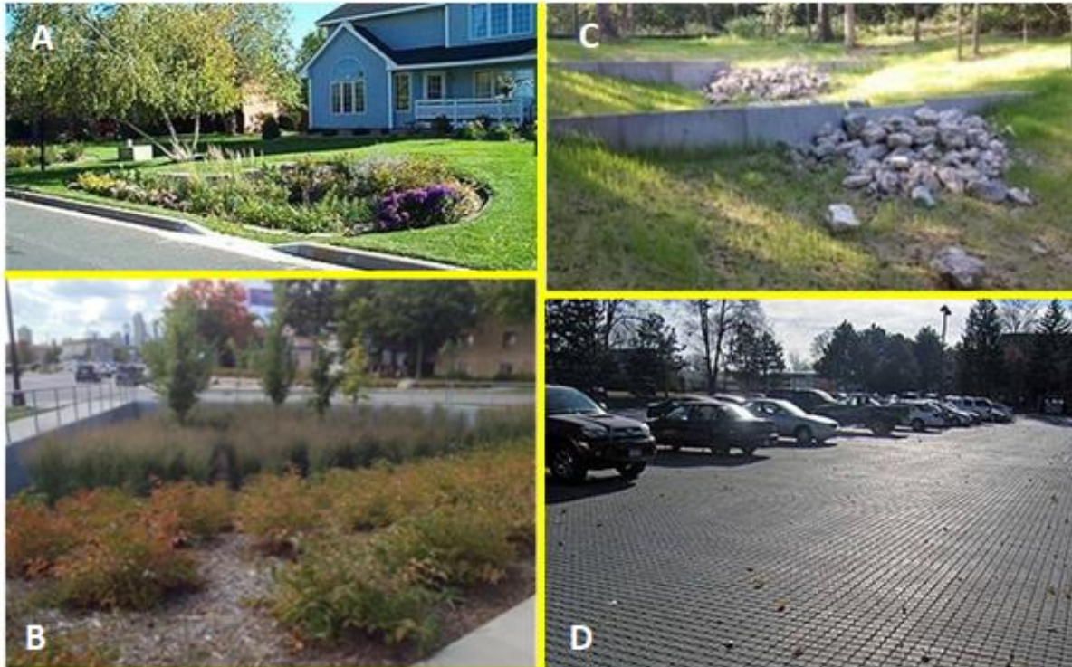
Figure 7: Examples of infiltration SCMs. From top to bottom: bioinfiltration, infiltration basin, swale with check dams, and permeable pavement (concrete pavers).
