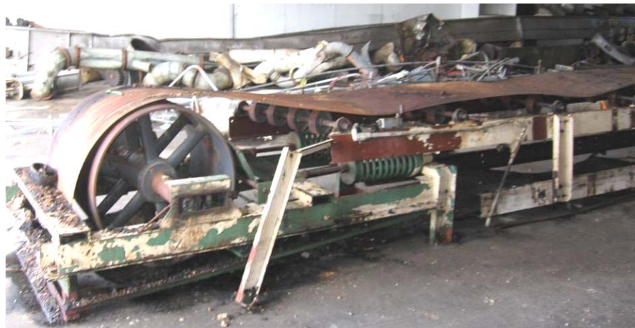
Figure 9. Silo tunnel steel conveyor belt (removed after incident)
