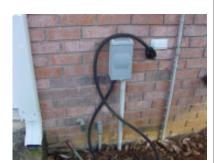
Figure 17. Large cord and plug to connect house transfer switch to PTO generator.
