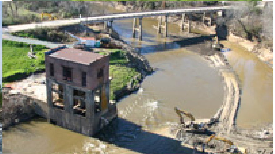
Carbonton Dam removal
