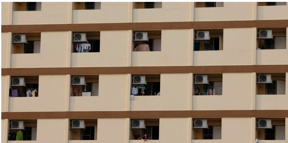
Different AC OU air flow arrangement
