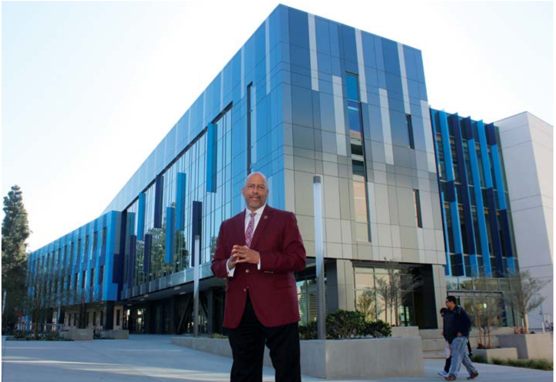
Cal State Dominguez Hills President Thomas Parham is pictured with the university's new, state-of-the-art science and innovation building. The three-story, 91,000-square-foot facility includes teaching and research laboratory space for chemistry, biology, physics and the Center for Innovation in STEM Education, including a maker-space fabrication lab. (Photograph by Brandon Richardson)
