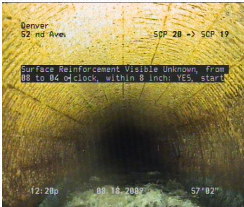
Corrosion in concrete pipelines
