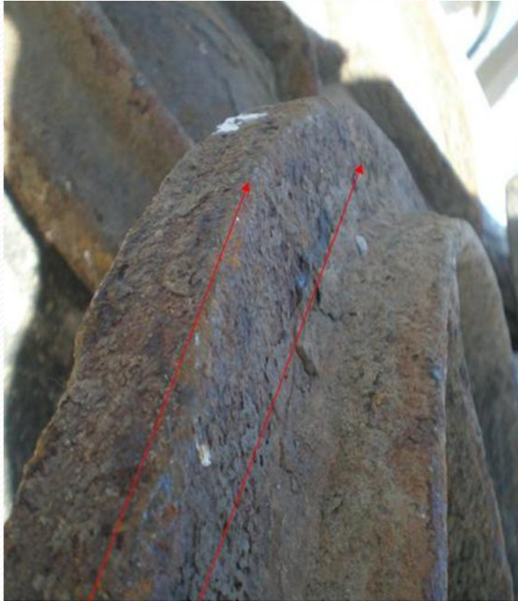
Corrosion of metallic manhole frame & cover
