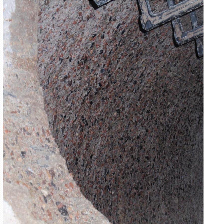
Corrosion in concrete manholes
