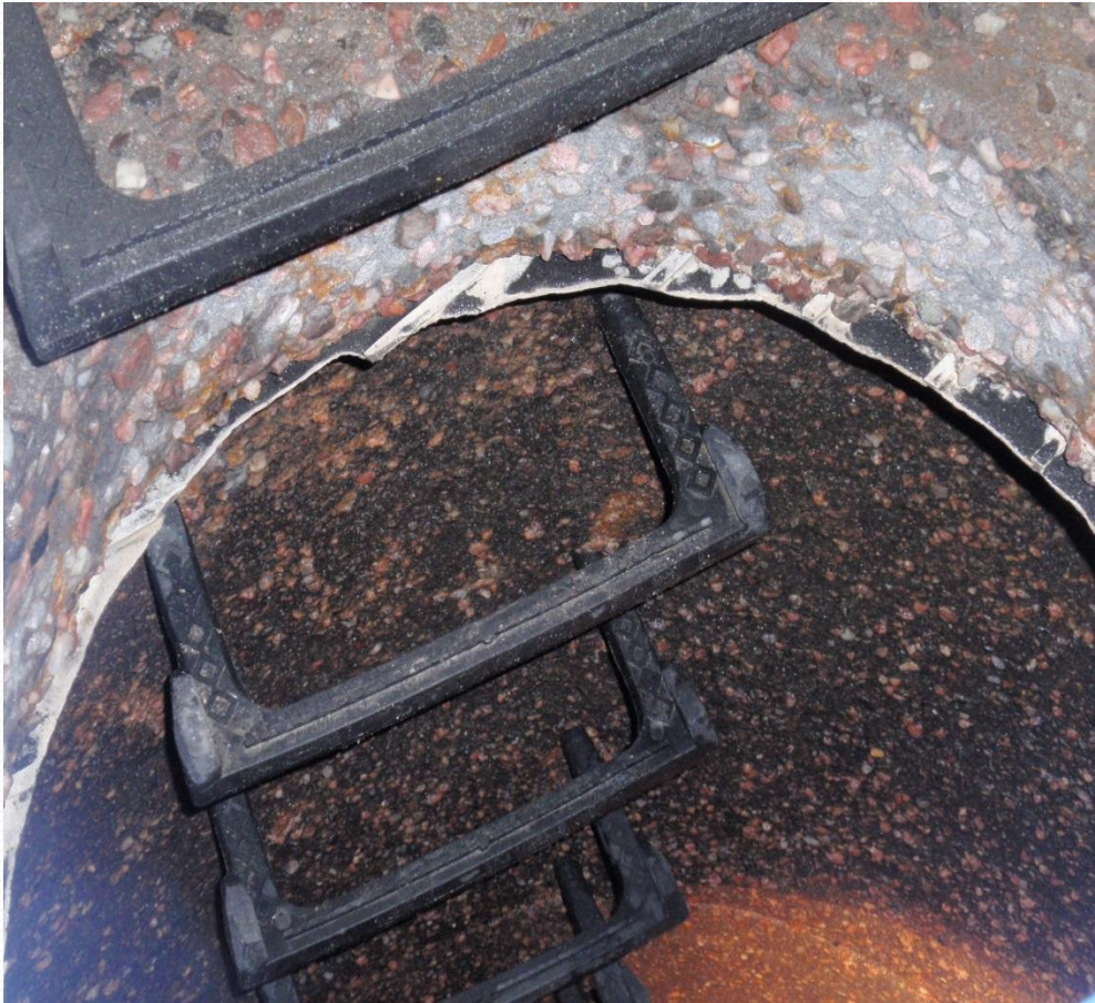
Corrosion in concrete manholes
