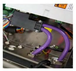
Figure A-58: J-Box Enclosure PROFIBUS Cable Routing
