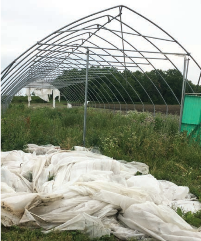
High winds ripped the poly off this high tunnel.
