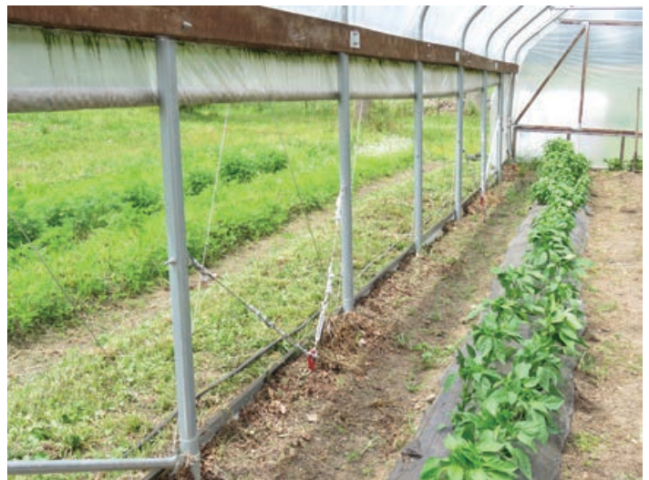
This moveable high tunnel is held in place by cables and turnbuckles connected to ground anchors. Peppers (foreground) and basil are thriving.
