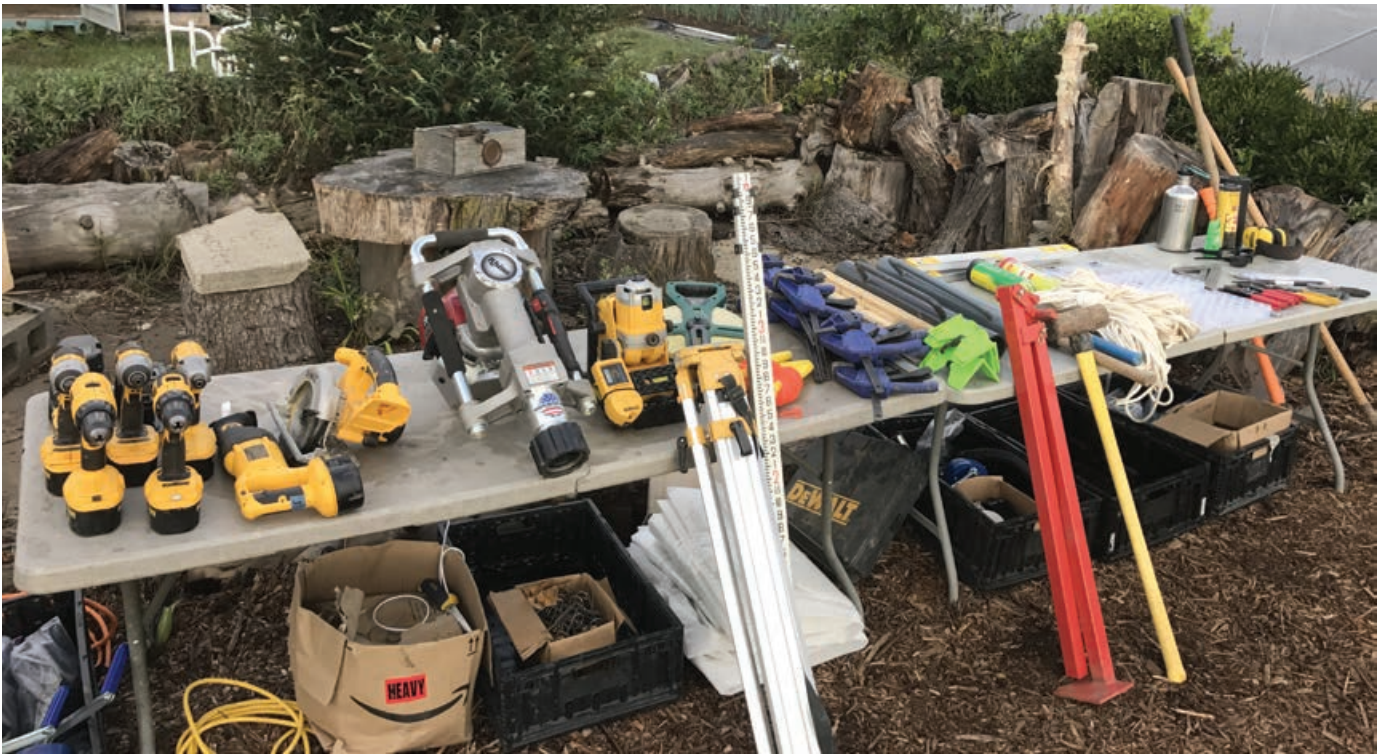
This photo from a high tunnel build highlights the many tools and supplies that are needed to construct the tunnel's infrastructure.
