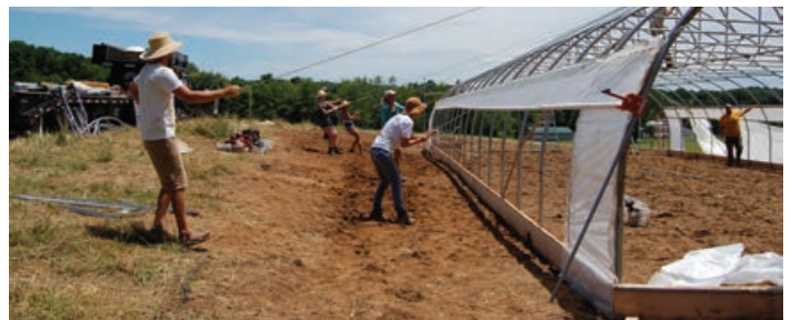
These photos highlight a high tunnel build at Harvest Moon Flower Farm. Many hands are needed, particularly when it's time to pull and fasten the poly into place.
