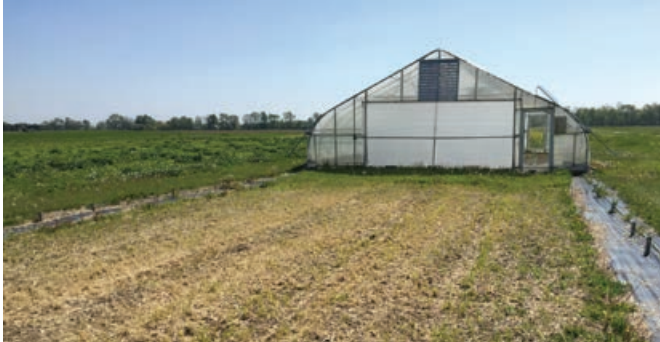
This high tunnel has a rail system frame with wheels at the base of its bows. The wheels rest on a rail, which the owner can roll it on.
