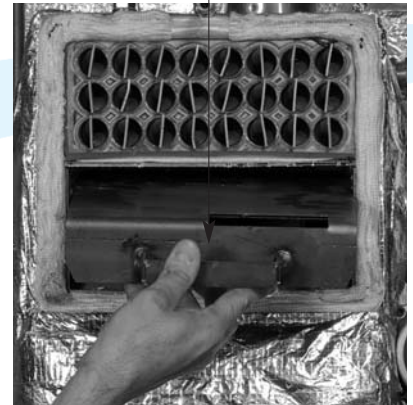
Figure 4-7: Removing baffles from boiler shell
