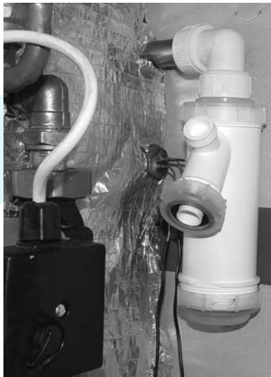
Figure 6-3: Condensate trap
