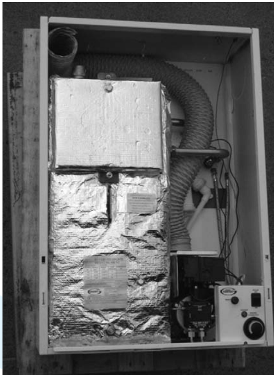
Figure 5-3: Grant Condensing Wall Hung boiler with front casing removed
