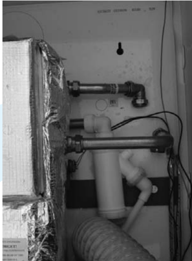
Figure 5-1: Non-system boiler flow and return connections
