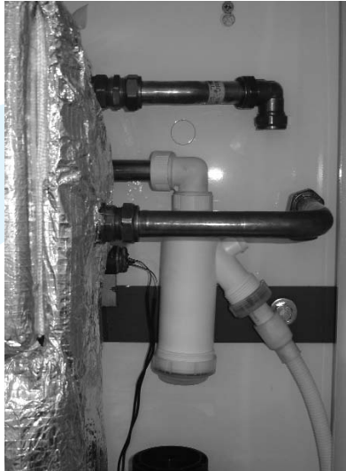
Figure 4-12: Re-fitting condensate trap
