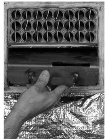
Figure 10-1: Removing the baffles
