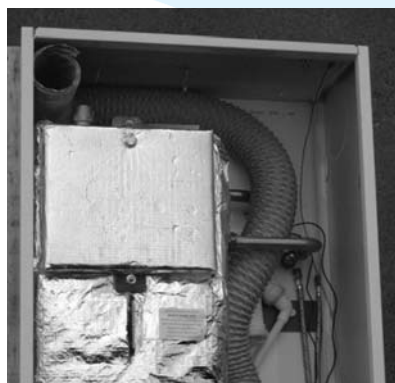
Figure 4-2: Dismantling the boiler
