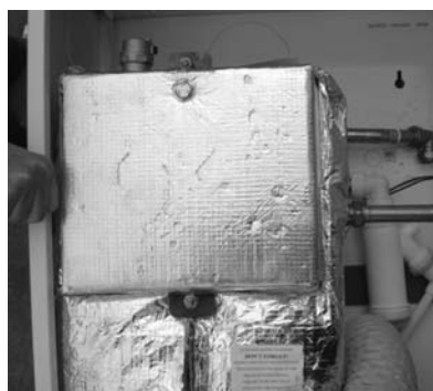
Figure 4-10: Re-fitting flow & return pipe
