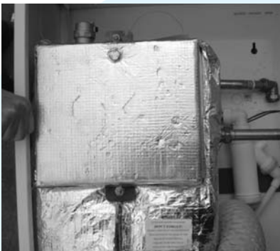
Figure 4-4: Removing flow & return pipe
