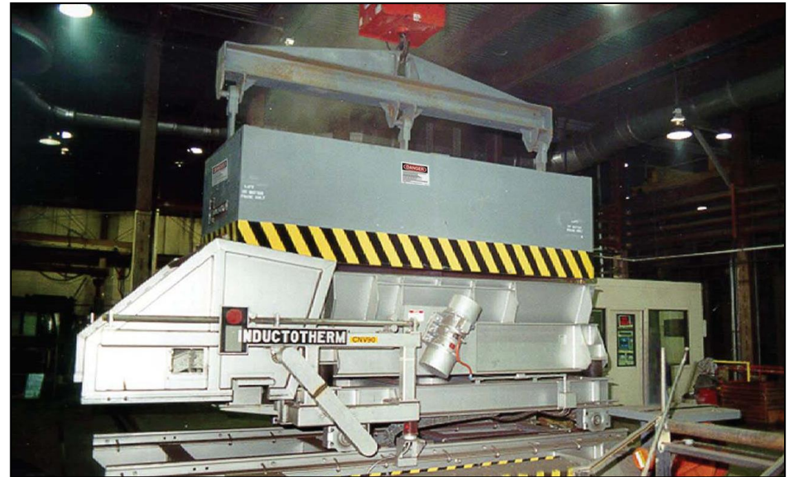
A charge bucket carried by an overhead crane drops its charge into a charge car
