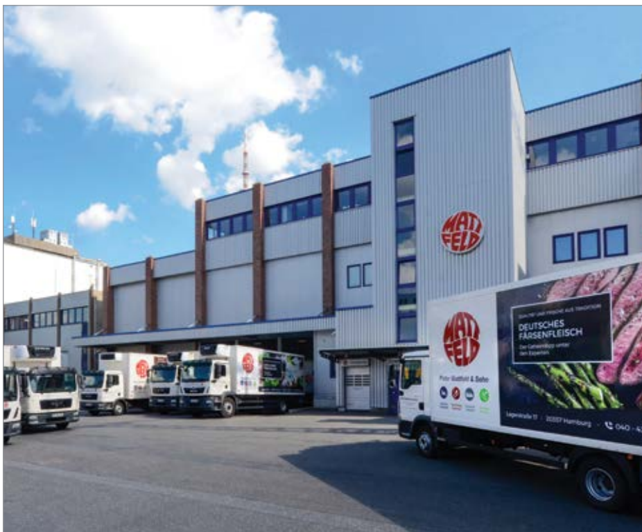
Peter Mattfeld & Sohn GmbH's plant in Hamburg, Germany.
