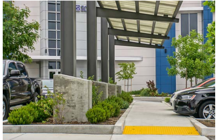
Landscaped islands provide clear pathways to primary building entry while minimizing pedestrian conflicts with vehicles.
