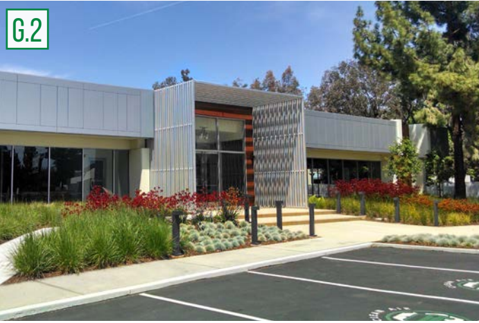
Changes in height and massing provide variation and articulation. Vertical building elements break up what may otherwise be horizontal architectural composition.
