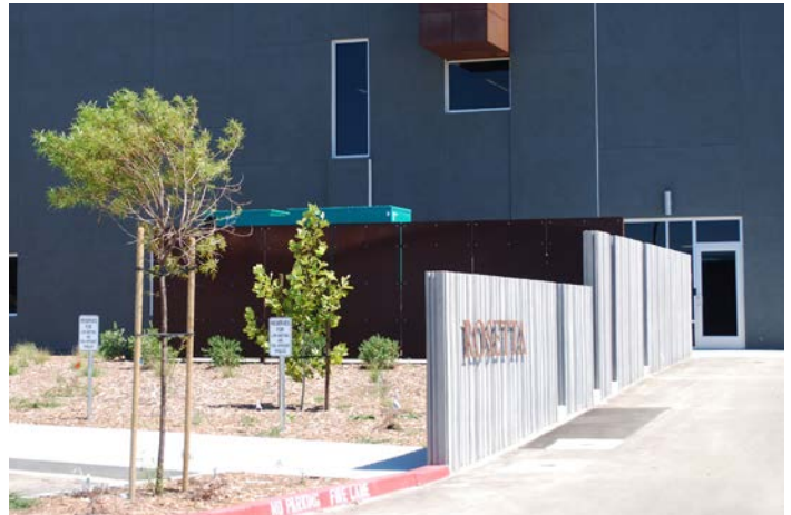
Wall and fencing designed as integral part of a site through continuation of building materials, with landscape minimizing visual monotony.
