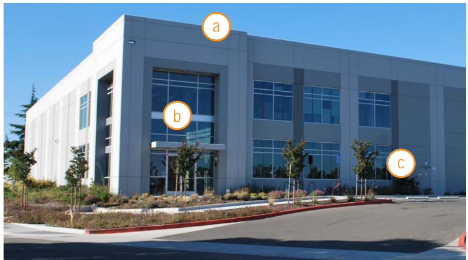
Current massing and articulation of industrial development.
