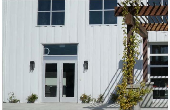
Light fixtures mounted at appropriate height for setting adjacent to building entry and shielded downward.
