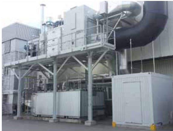
Single-bed RTO with concentrator
