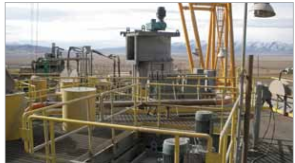
Media Retention Screens
