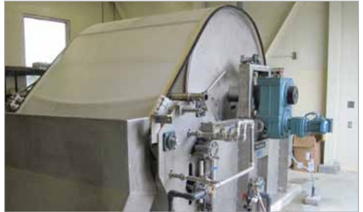
Drum Belt Vacuum Filter
