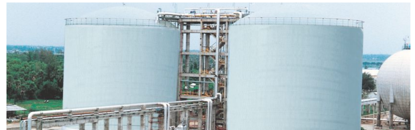
Cryogenic Ammonia Storage Tanks with associated facilities
