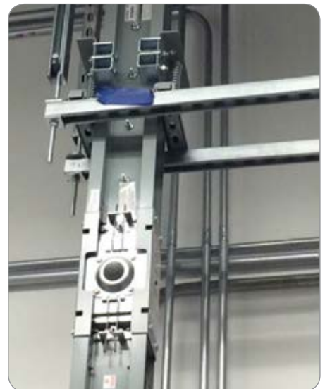
Complete outdoor run of Spectra Series Busway
