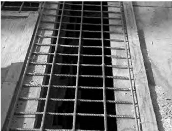
Figure 12 – Mesh used as fall protection on wall pour
