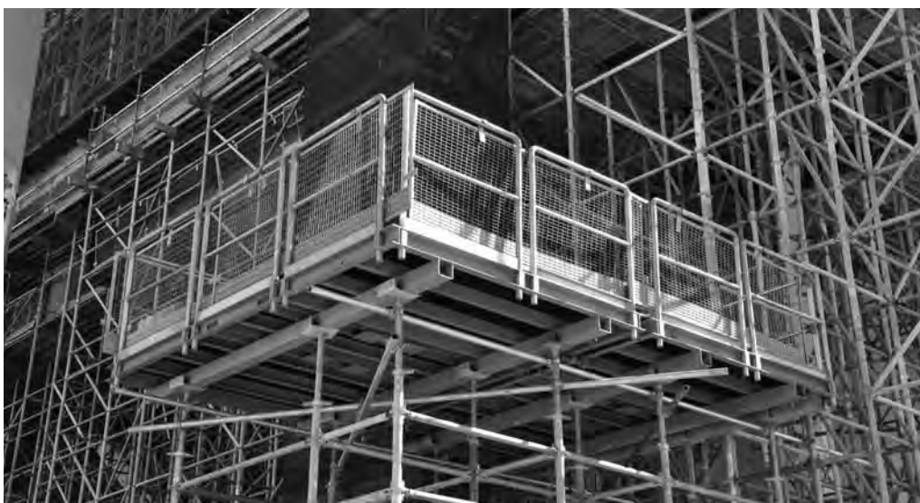
Figure 7 – Engineered loading bay.
