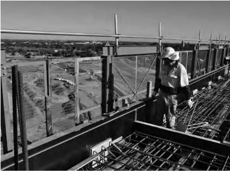
Figure 6a – General view
