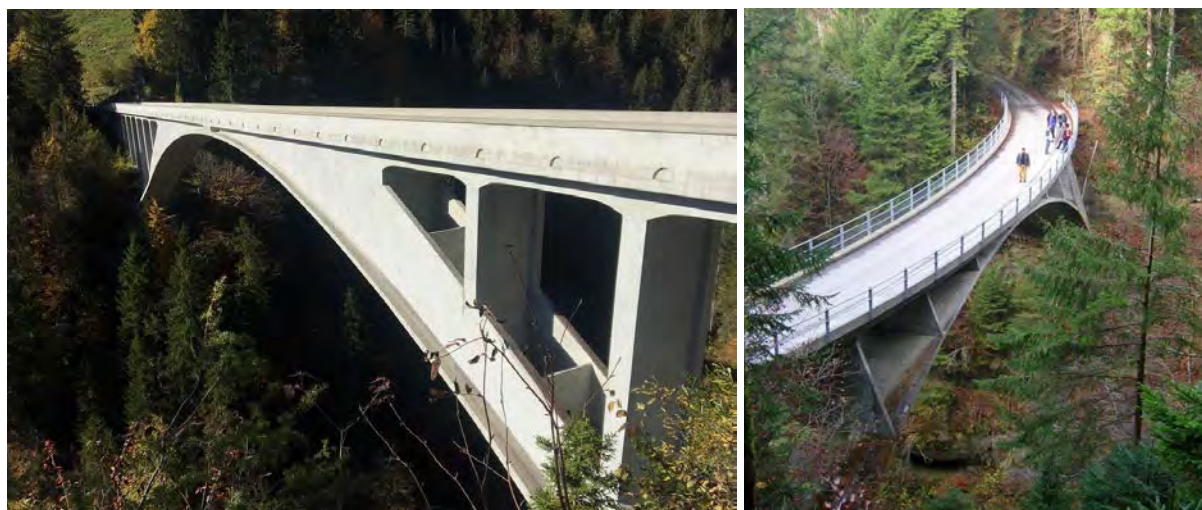
Figure 7. Robert Maillart’s contrasting concrete arches at Salginatobel (left) and Schwandbach (right).
