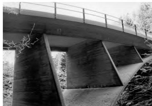
Figure 3: The Schwandbach Bridge, trapezoidal vertical cross walls
