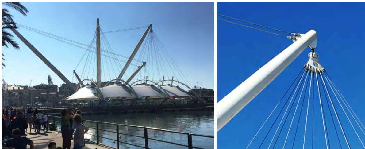
Figure 5. Bigo's structural elements are all exposed, and clearly display the load path.
