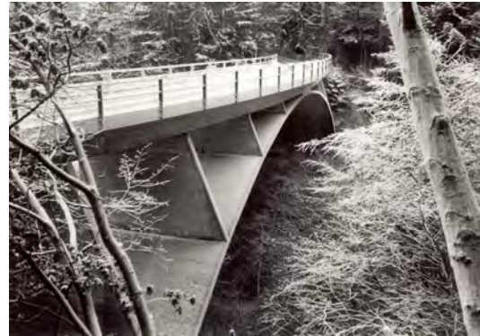
Figure 2: The Schwandbach Bridge, near Hinterfultigen, Switzerland, built in 1933
