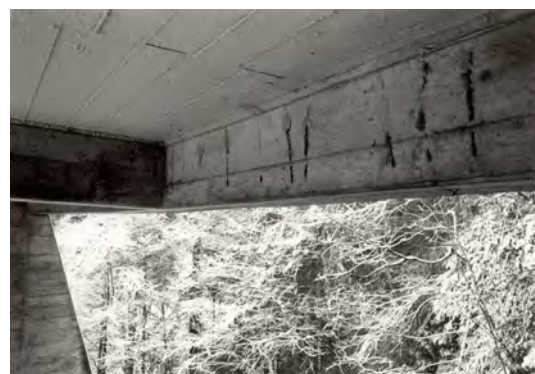
Figure 4: The Schwandbach Bridge, beneath the deck
