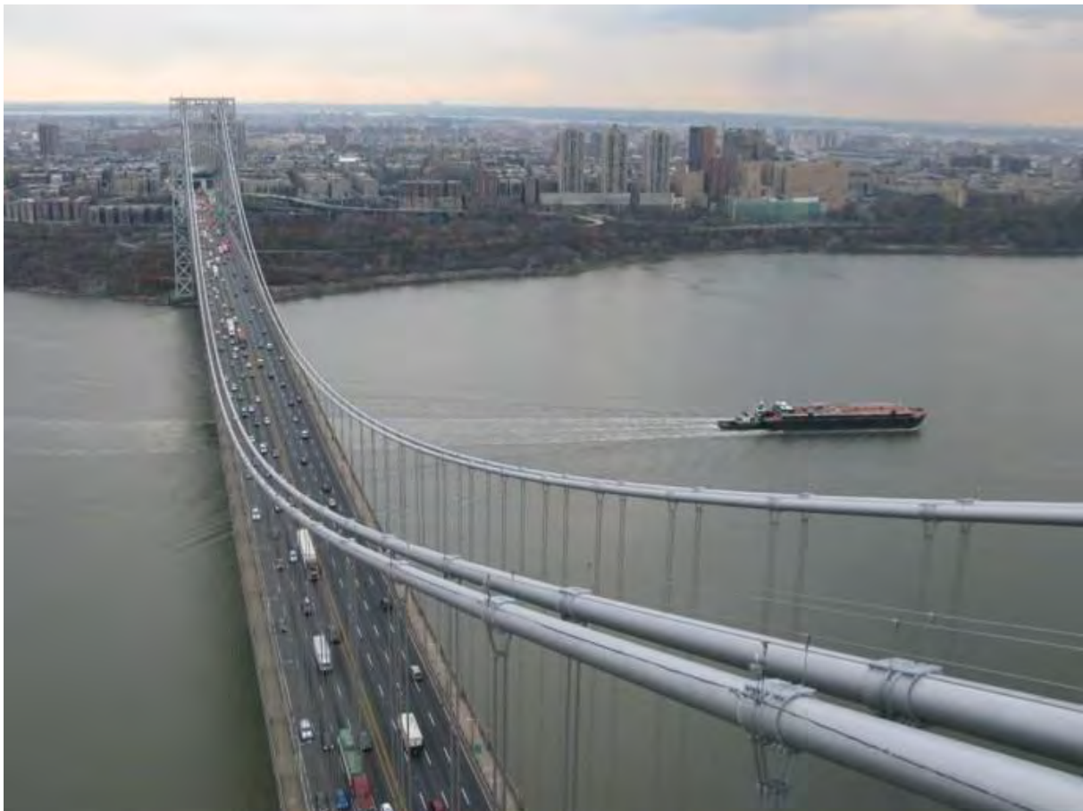
Figure 1: The George Washington Bridge (New York, USA)
