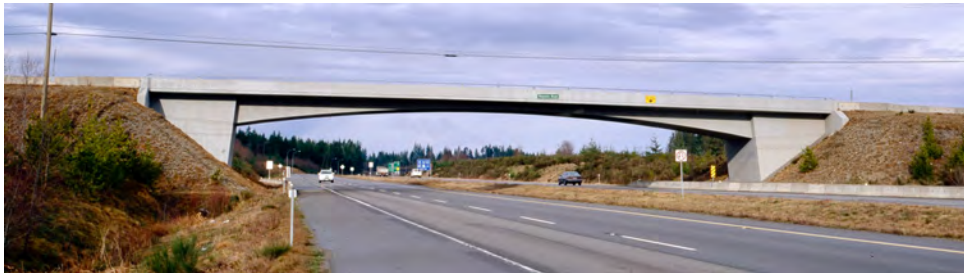
Figure 2: Royston Road Underpass, British Columbia, Canada
